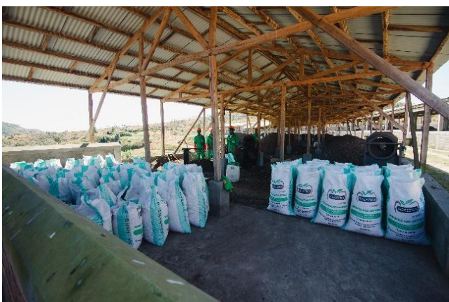
Figure 1 : Drying system and storage conditions of fecal sludge at the Fianarantsoa treatment site
